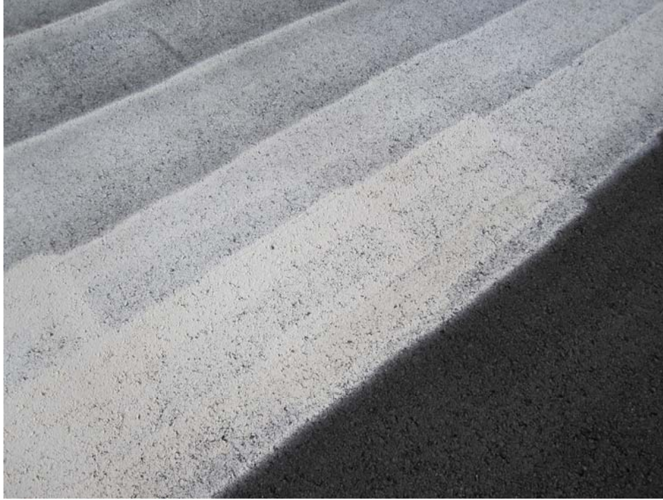
R0826AGR-25. Satisfactory Paint.
