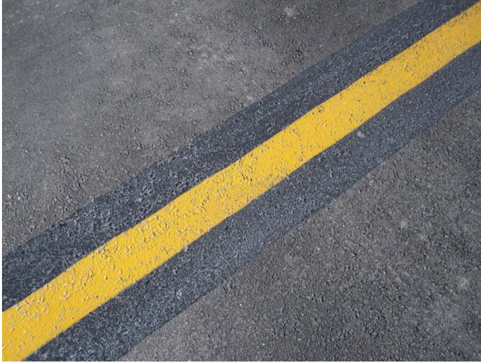
TEAGR-30. Satisfactory Paint.
