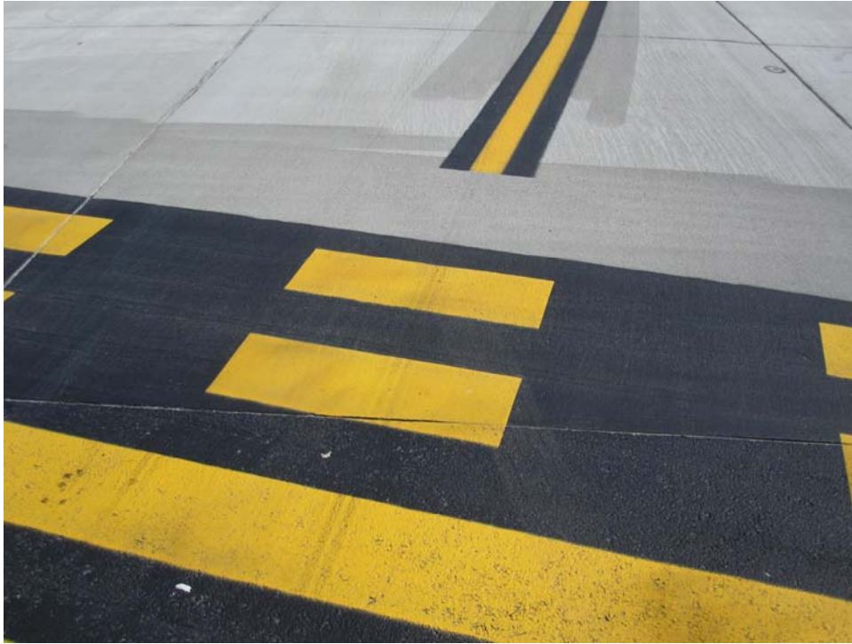
TCAGR-40. Satisfactory Paint.
