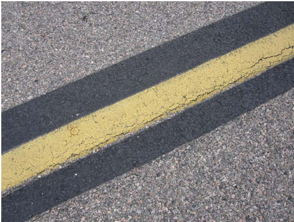
TCAGR-20. Satisfactory Paint.
