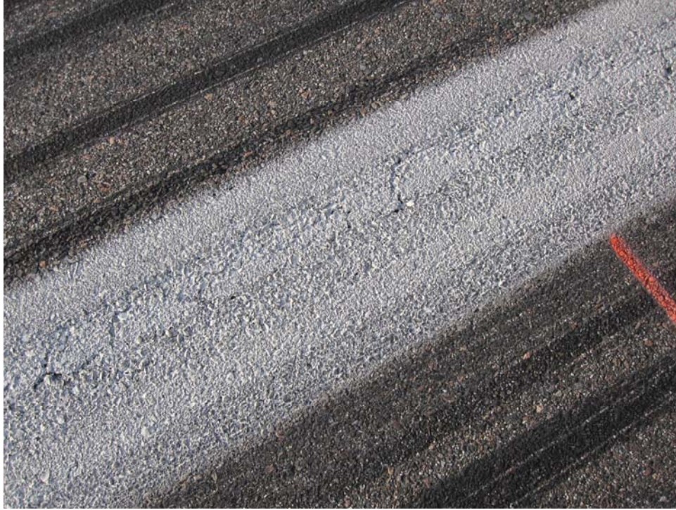
R0826AGR-30. Satisfactory Paint.
