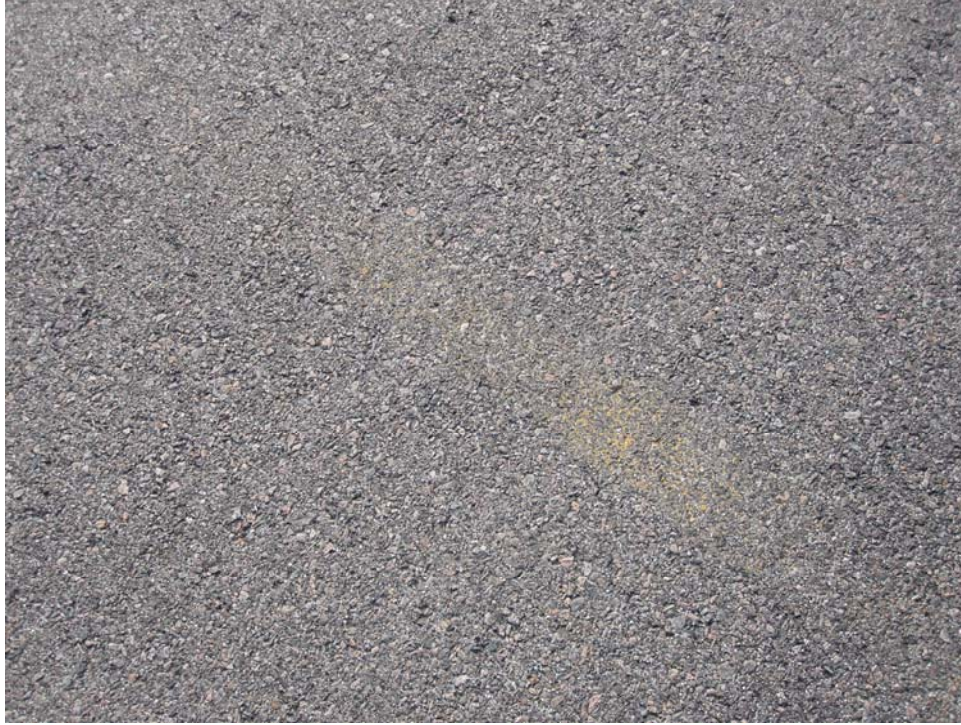
A01AGR-50. Unsatisfactory Paint.
