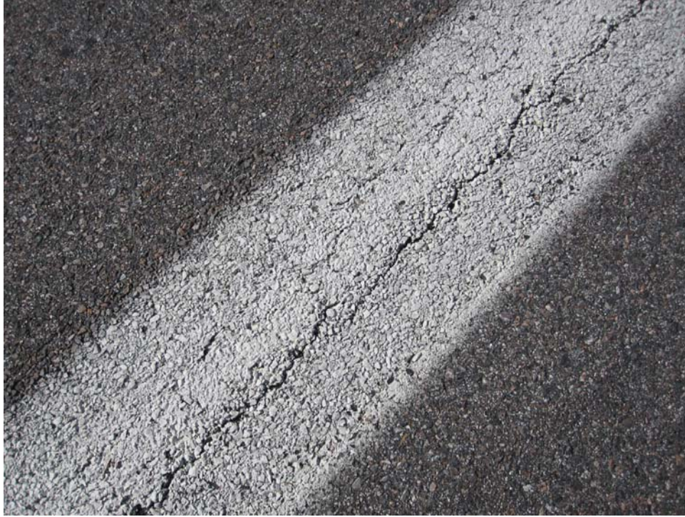
R0826AGR-20. Satisfactory Paint.
