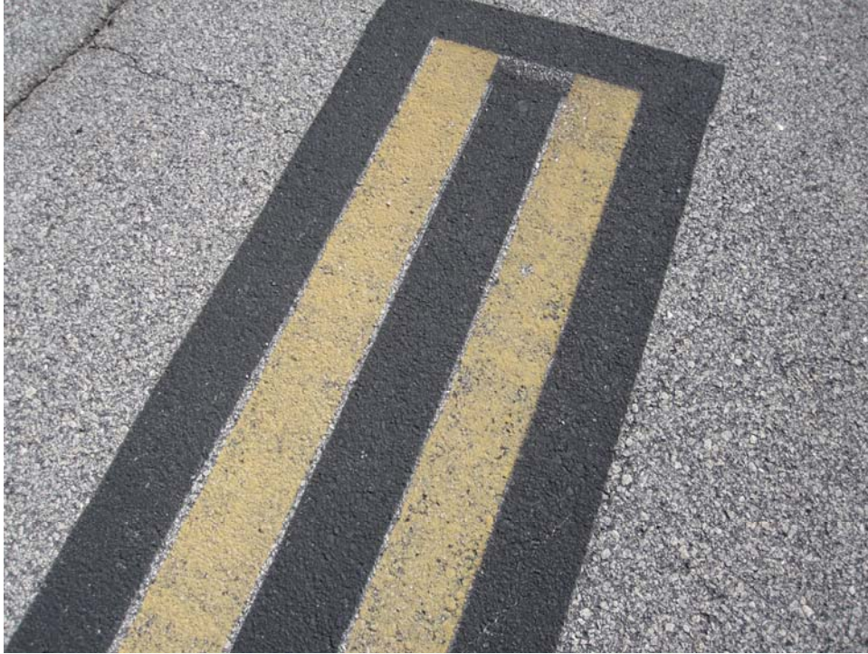
TCAGR-10. Satisfactory Paint.
