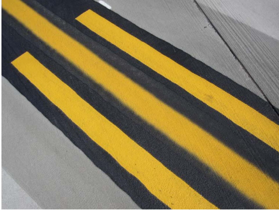
TAAGR-10. Satisfactory Paint.
