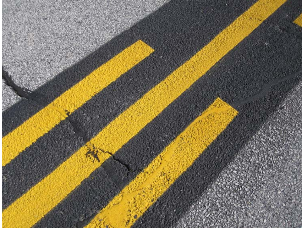
TEAGR-10. Satisfactory Paint.
