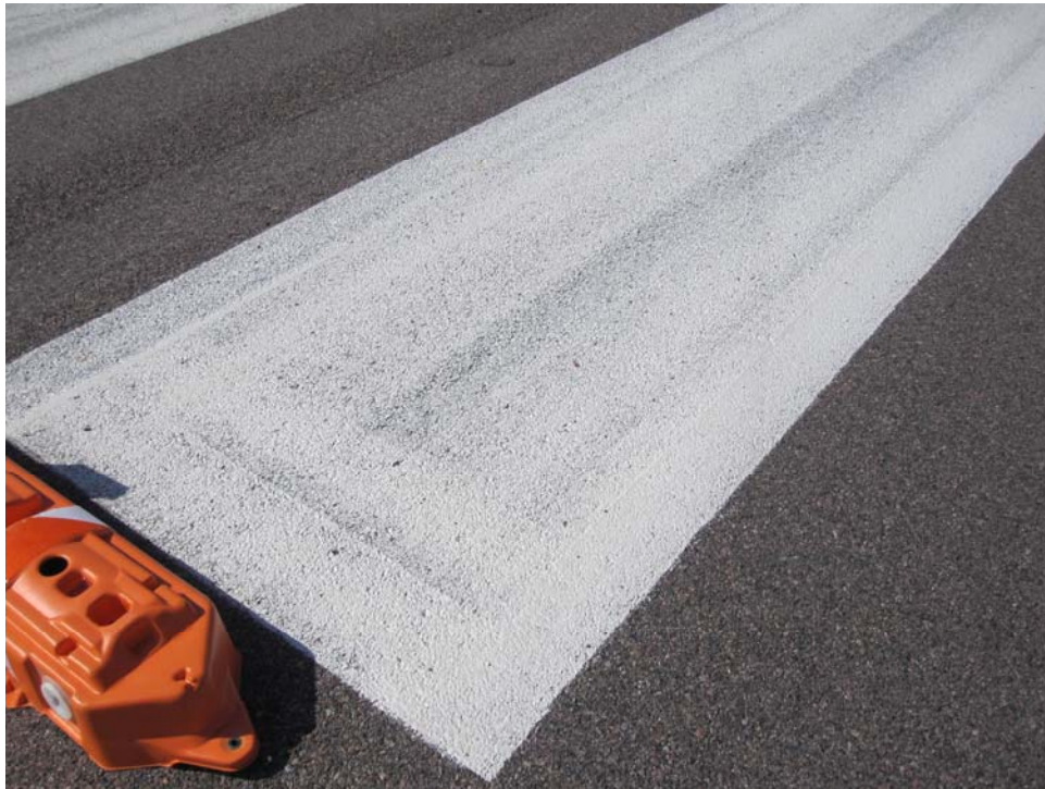
R0826AGR-10. Satisfactory Paint.
