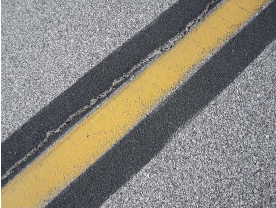
TAAGR-20. Satisfactory Paint.
